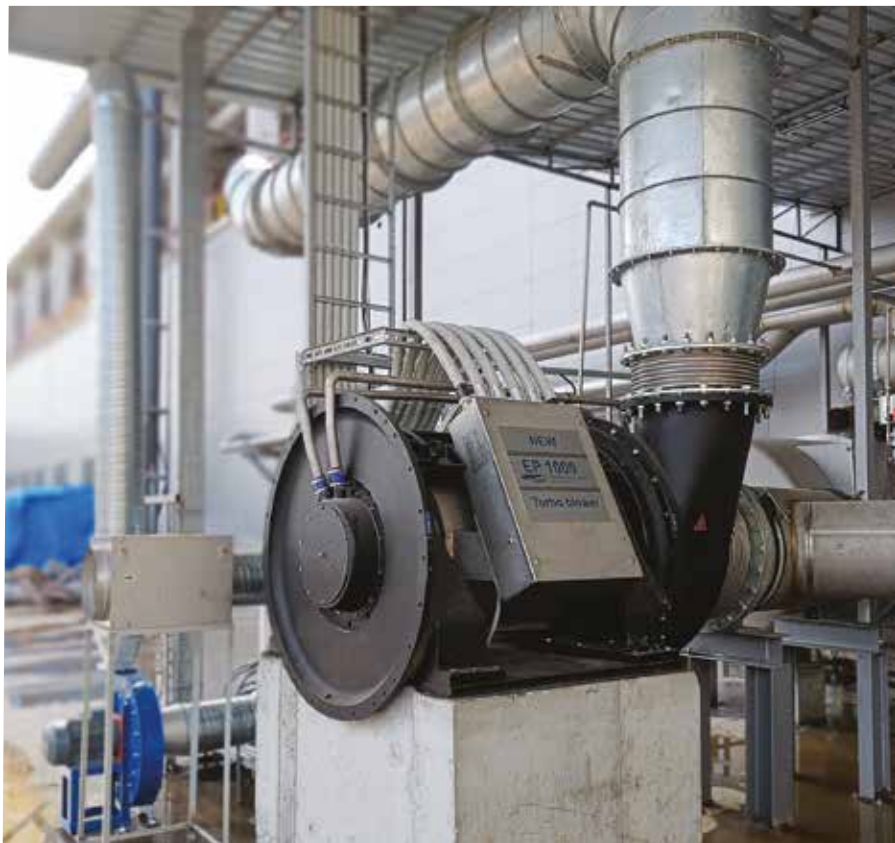
Image 1: TRunEcoEP1000.jpg: RunEco EP1000 Turbo Blower with Active Magnetic Bearings.
