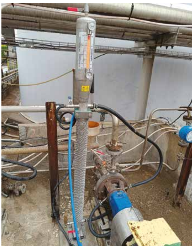
Image 1: (Left) SZ8 SealCooler system installation.
