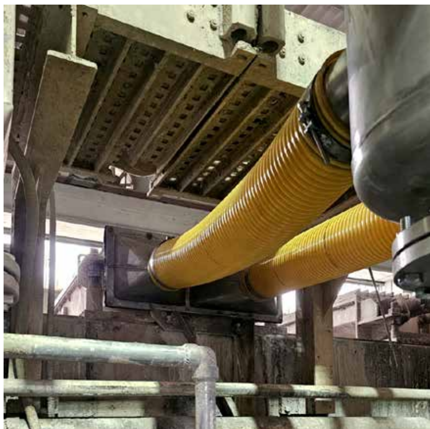
Image 7: New Duoflow separators downstream of the dandy roll.
