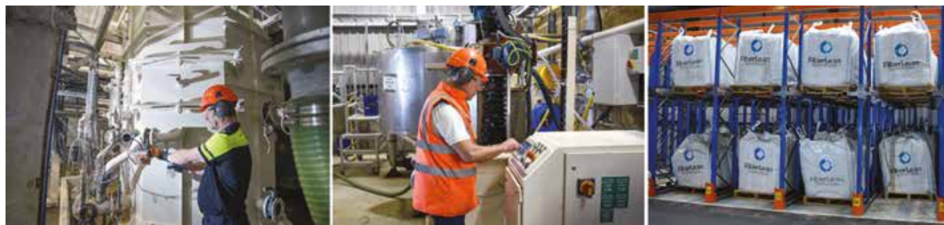
Figure 10: FiberLean Technologies Limited MFC production facility in Cornwall, UK.
