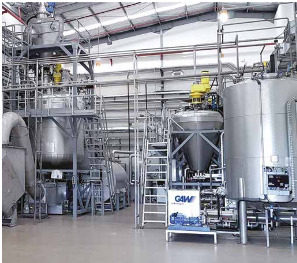
Image 3: An industrial demonstrator unit is in operation since 2021.
