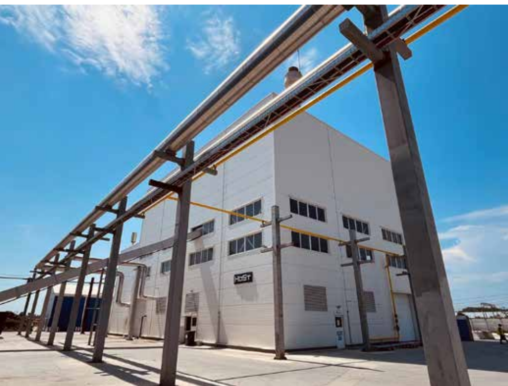
Figure 4: Exterior of the CHP plant.
