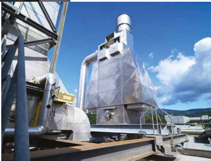
Image 4: At the Gernsbach mill, waste heat from the TURBAIR® system is reused to preheat air and warm process water. ©Raphael Zubler / Everllence
