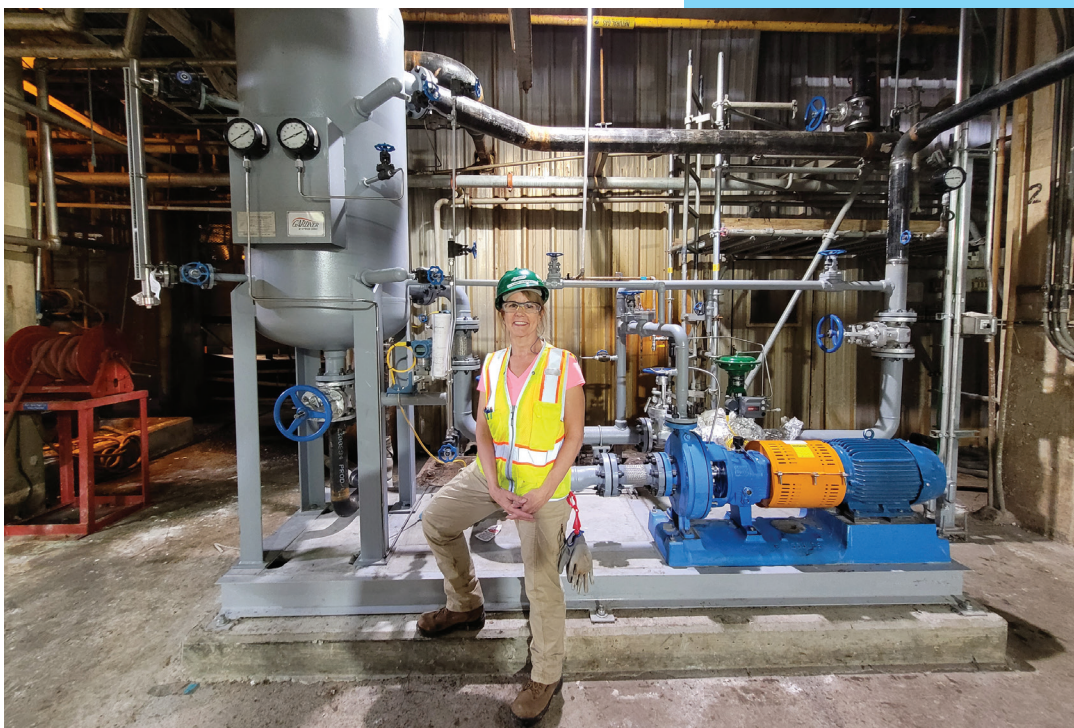
Figure 3: Lisa Freed, of Deublin Company, in front of a newly installed separator skid.
