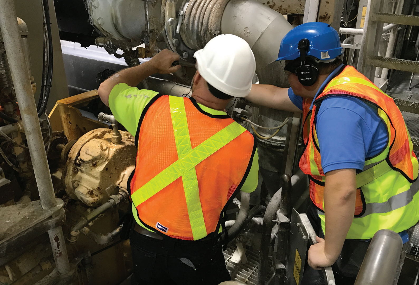
Image 1 (Left): RunEco EP Turbo Blower with active magnetic bearings.
