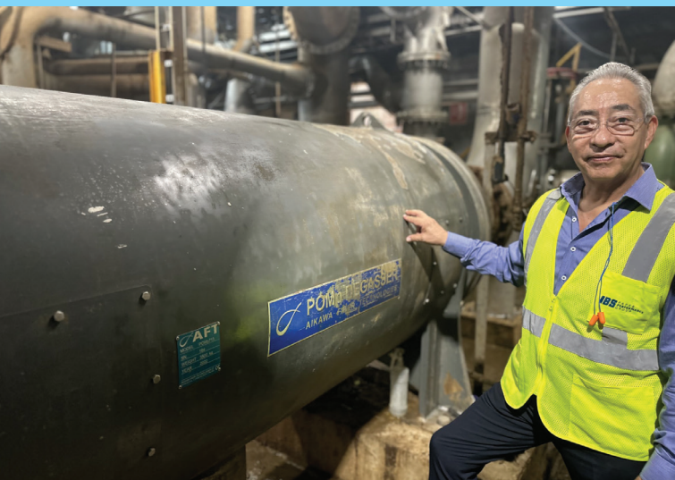
Figure 5: “With a POMp Degasser, you enjoy the extreme absence of air in your process. This accomplishment is the foundation for consistent high quality at increased speed, delivering increased strength to the boxes of our customers,” says Mario Ramirez,
