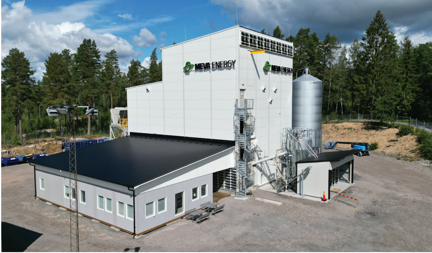
Figure 4: Meva Energy's thermochemical conversion technology converts biogenic residue, including sawdust, to renewable gas. The gas can then be used to fuel power generation or to replace fossil gas consumption in industrial heat systems.
