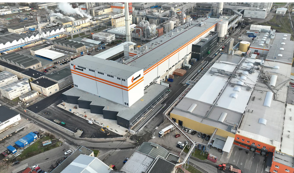
Figure 4 & 5: The deep-channel high-bay warehouse, with its high storage density, enabled Mondi Štětí to locate an automated storing and sorting buffer directly after the production line, despite the confined mill layout.
