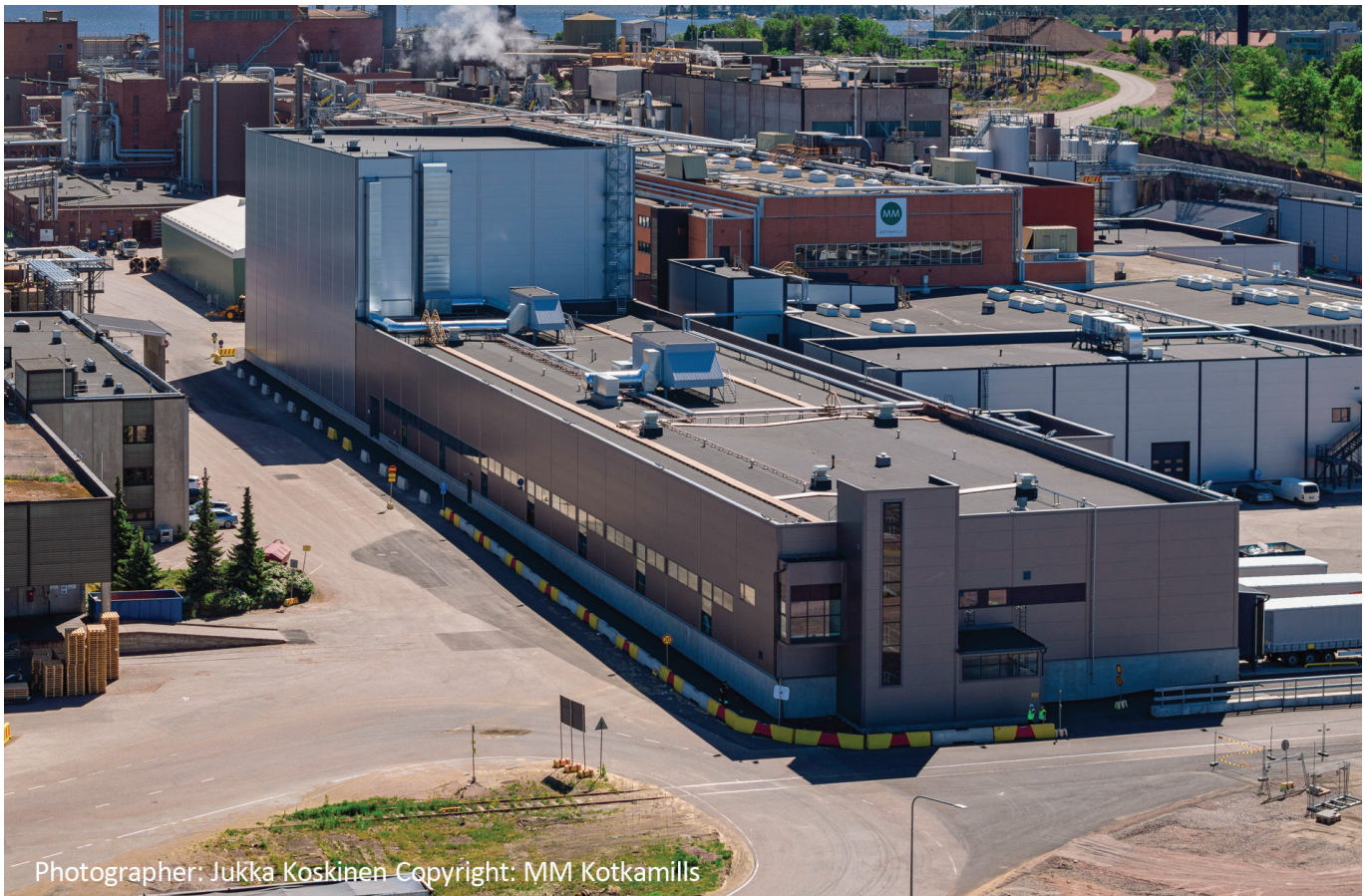
Figure 8: For MM Kotkamills, the centralized automated high-bay warehouse enabled the sheeting function to operate in parallel with production.
