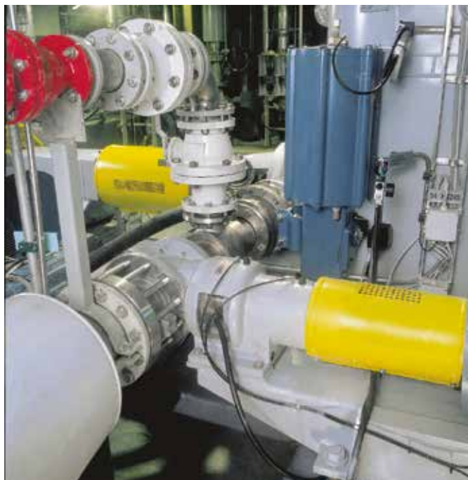
Figure 23: ClO 2 mixing with chemical mixer.
