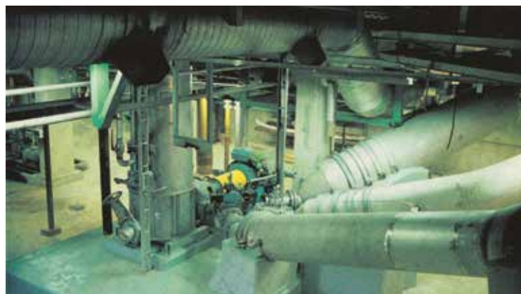
Figure 12: Stock flow splitting with MCE pump and flow divider into three storage towers.
