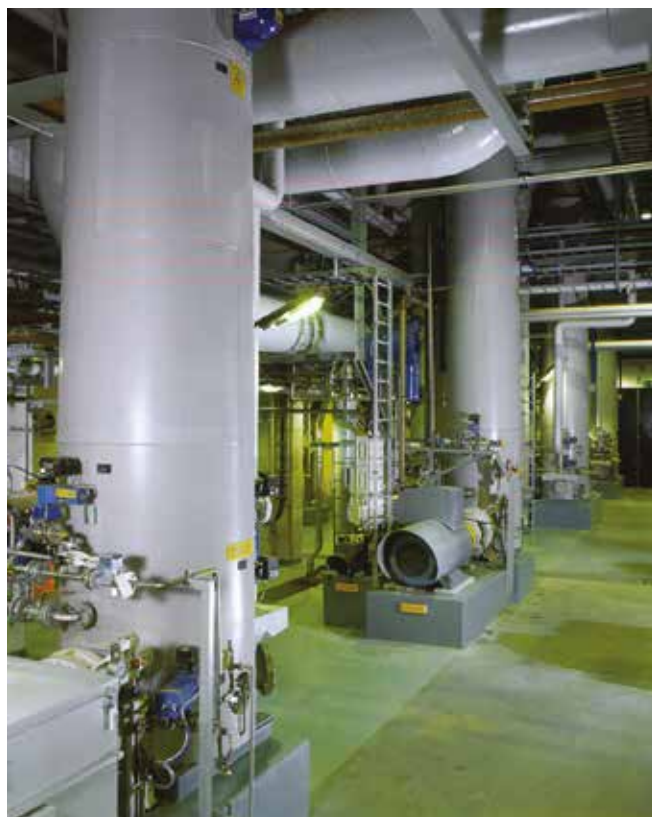
Figure 8: Typical MC pumping arrangements. The stock level in the MDL dropleg is measured and controlled, thus providing constant operating conditions for the pump.
