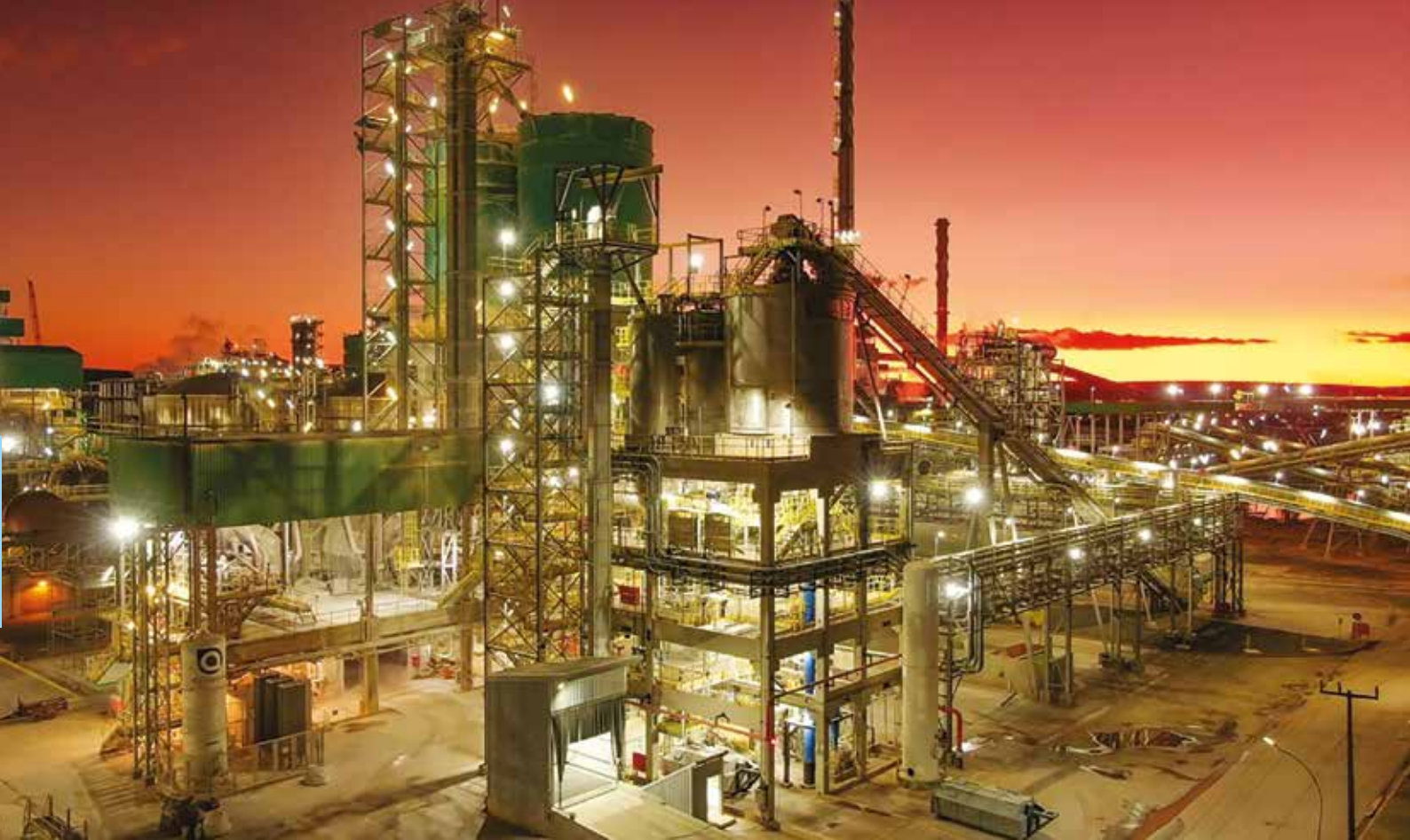
Figure 1: ANDRITZ gasification plant for the lime kiln.
