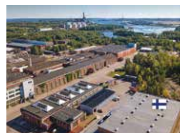
Karhula Plant: Rolls, Covers & Vacuum Pumps.
