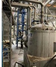
A new AFT fine screening line started in 2020. Multiple stages of screening are a proven approach to increasing quality and minimizing fiber loss.
