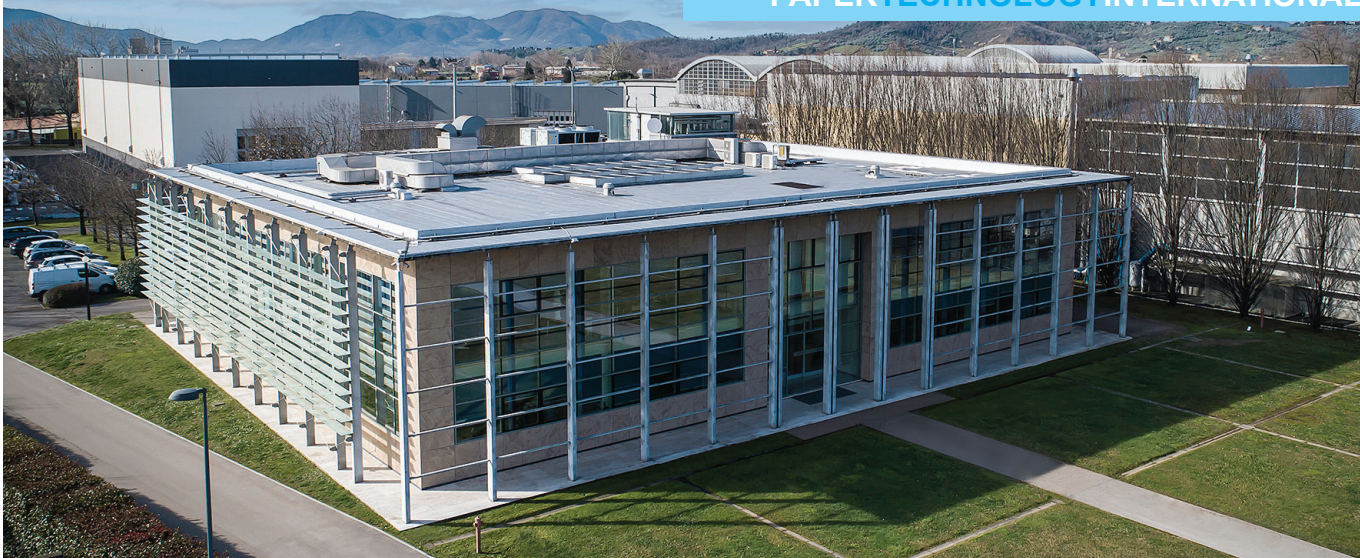
Figure 7: Toscotec's headquarters office building in Lucca, Italy.
