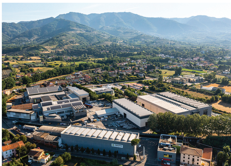
Figure 1: Toscotec's headquarters in Lucca, Italy.
