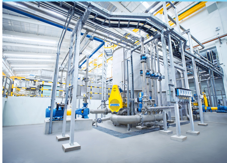
Figure 8: Stock blending system as part of the stock preparation.
