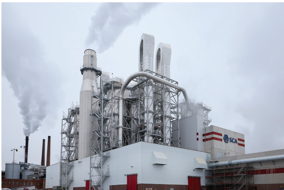
Figure 8: A newly erected building which houses dewatering, two twin roll presses, two flash dryers and baling, as well as a wrapping facility.
