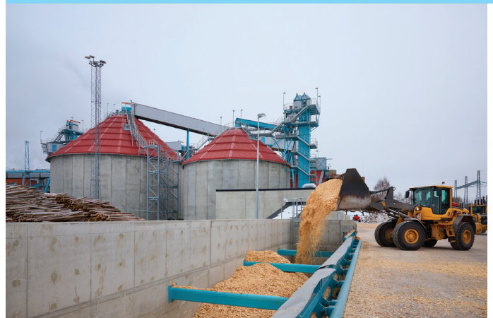
Figure 3: Wood chip silos and input of sawmill chips.
