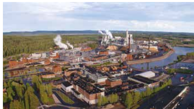
Figure 2: At all Metsä Board paperboard mills, water recycling is of the utmost importance.
