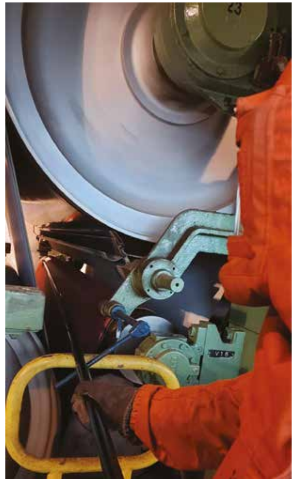
Figure 4: Pocket humidity levels are measured as a part of the drying section audit.
