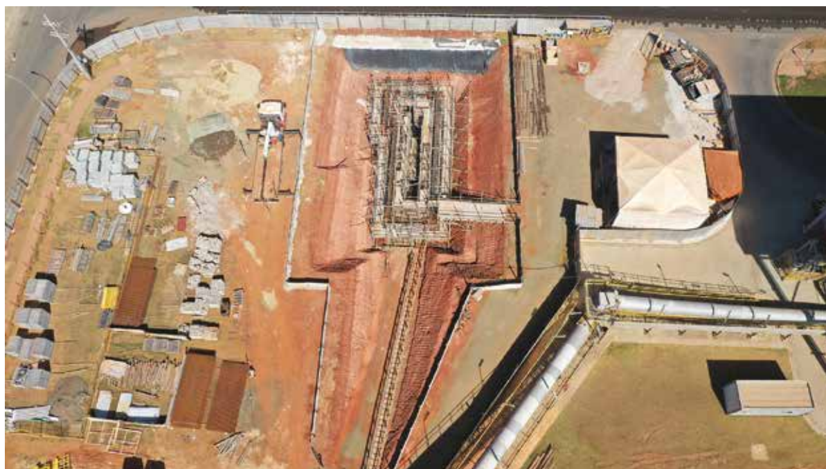
Figure 1: Status of the on-site construction works in May.
