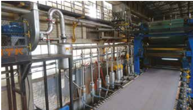
Figure 1: Overall vacuum system layout with drainage elements and wire before start-up.
