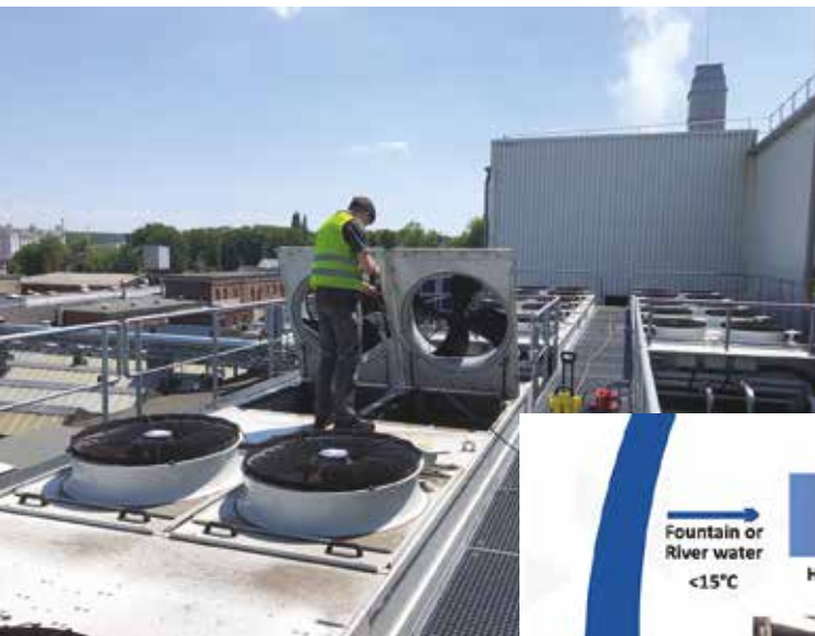
Figure 5: Dry coolers feature openable fans to enable cleaning
