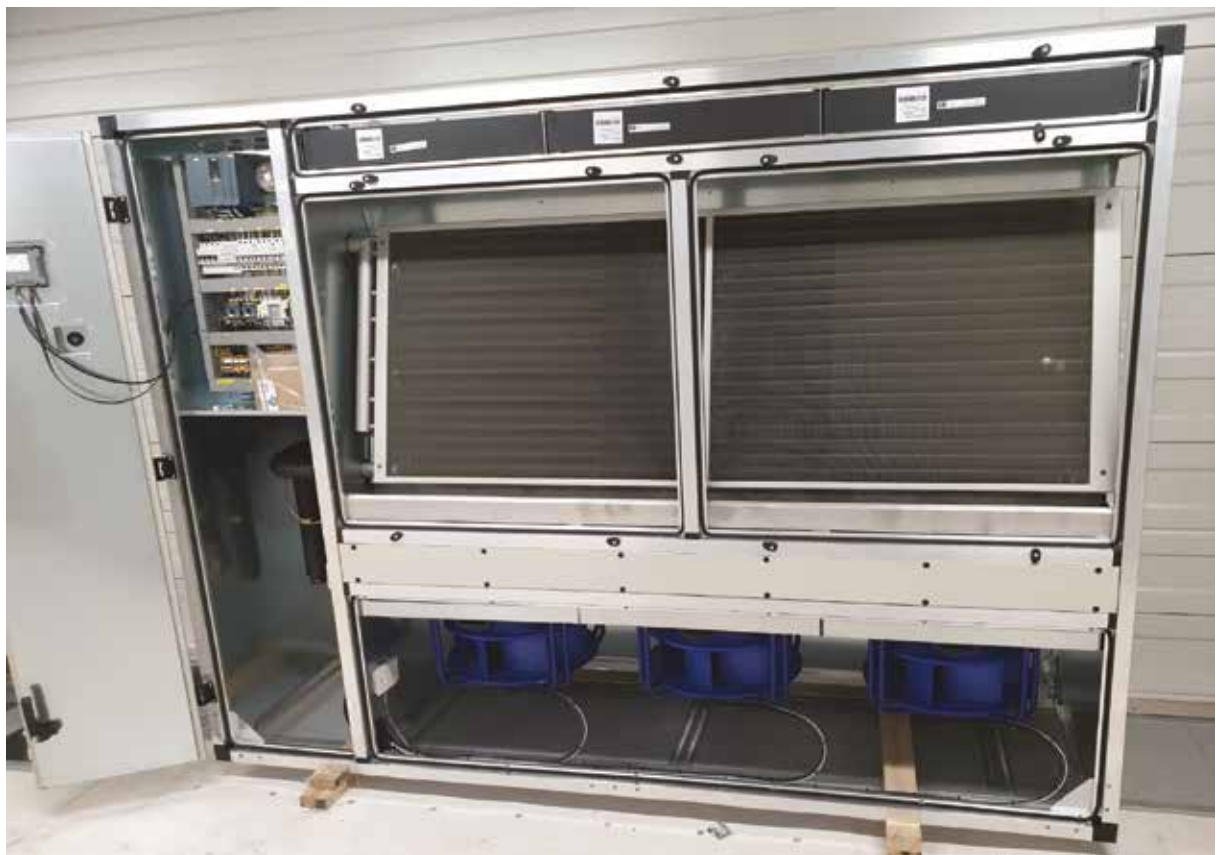
Figure 3: Specially engineered climate cabinet, A-shape coil and Siemens S7.
